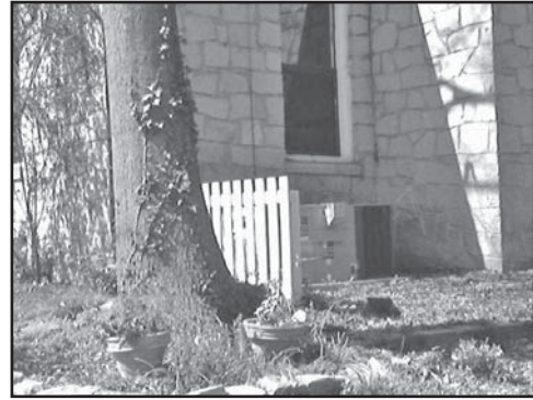
This HVAC system is properly screened by a picket fence. The addition of plantings would make this an ideal screening of this HVAC unit.
