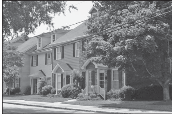
This multi-family development in Gainesville, Georgia utilizes a stoop entry and porch supports found within its area of influence, as well as a simple entablature and modest gabled roof. The windows are also in keeping with its area of influence. It is important that multi-family housing be compatible in scale and detailing within its area of influence.
