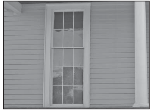
This six-over-nine light floor-to-ceiling window is one of the few examples of this type of window in Kennesaw. During the rehabilitation of this property for use as an office the window was appropriately retained.
