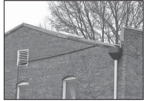
This gable-roofed building on Main Street utilizes a parapet wall to screen this gable from view, as well as to screen any equipment that could be placed on this roof.
