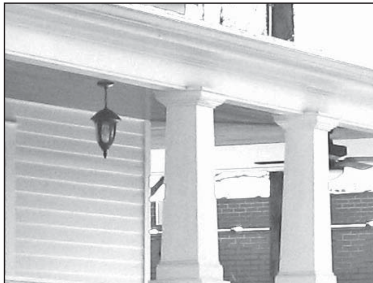
Pendant and other lantern-like lighting is appropriate to residential architecture within the district. Scale is of primary concern when choosing lighting for a residential building.
