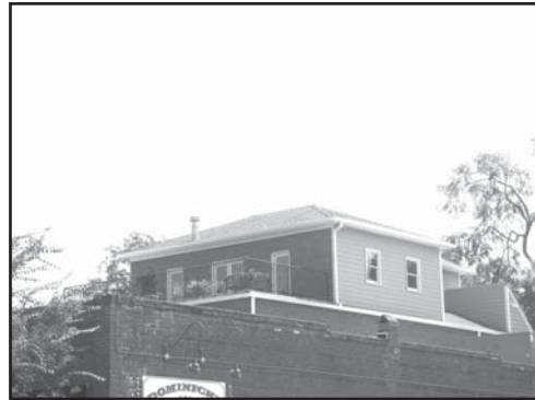
This rooftop addition in Norcross, Georgia, is appropriately set back from the front facade so that it is not seen from the public right-of-way. Additions must be stepped back from facades that can be seen from public rights-of-way.
