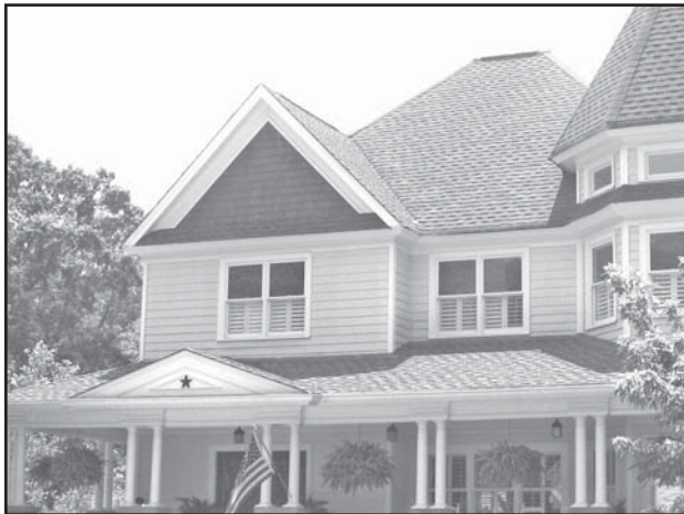
This residence in Norcross utilizes both hardiplank siding and cedar shingles to create architectural interest. The use of a variety of materials in new construction is encouraged.
