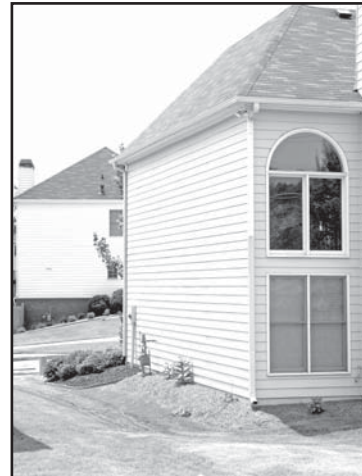
“Blank facades” are facades with no windows, doors, or architectural treatments. These facades are not permitted in the district.
