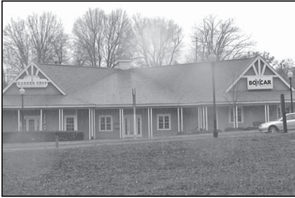
This commercial structure in Kennesaw, adjacent to historic residences and the commercial core on Main Street, utilized the massing and scale of the depot when it was designed. In doing so this building does not overpower the adjacent residential properties, yet still maintains a commercial feel.
