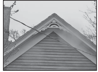
This verge board on this Victorian style cottage is a character-defining element of the style of the cottage and must be maintained and retained.
