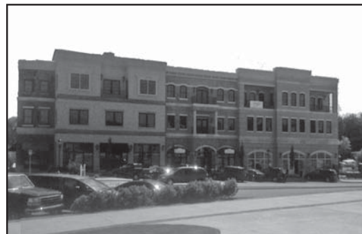
This building exhibits many qualities of a successful infill commercial building including conformity of materials and their use. There are distinguishable bases and cornices for each level of the building, and the building materials and facade articulation used provides architectural interest and variety to each facade.
