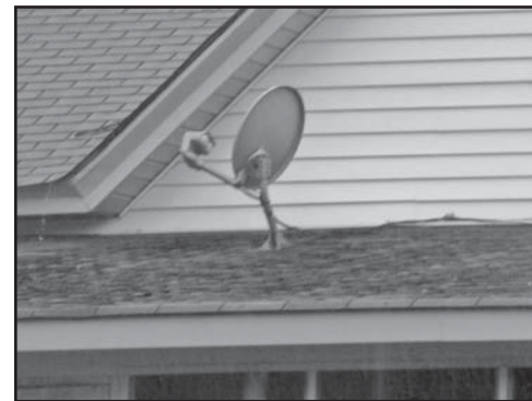
Satellite dishes must always be placed on the least visible facade from the public rights-of-way. The placement of such antennae's on a side, or rear, porch roof is often a good solution.
