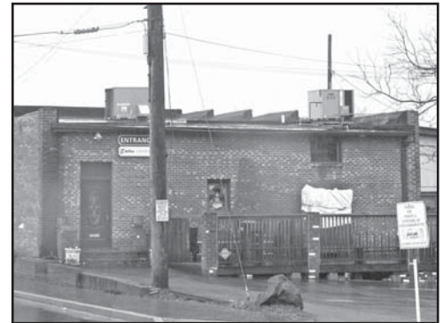
This gable-roofed building on Main Street utilizes a parapet wall to screen this gable from view, as well as to screen any equipment that could be placed on this roof.
