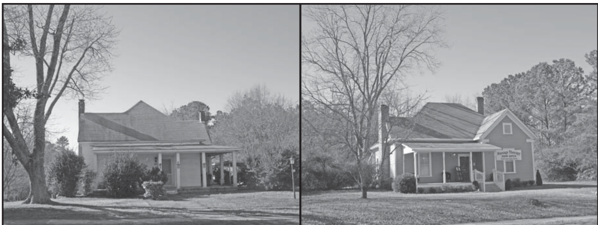
This pyramidal roof (left example) and the hipped roof (right example) and their gabled extensions are integral to the house type of these properties. Their alteration in pitch or form would impact the integrity of these homes.
