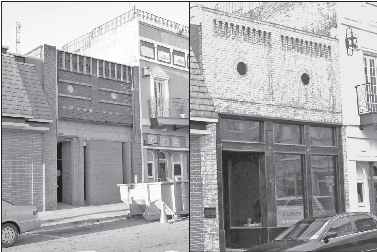
This building in Gainesville, Georgia, was poorly rehabilitated several decades ago when the storefront was infilled with brick (left). Thorough research and care in following the Secretary of the Interior's Standards for Rehabilitation have resulted in a recent rehabilitation that exhibits a historically appropriate storefront (right).
