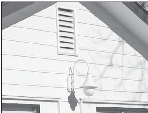
This contemporary fixture is appropriately scaled for residential use. If the proportions had been larger on this fixture it would not be appropriate for residential buildings in the district.
