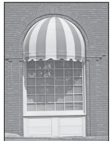
An arched awning for an arched opening like this is appropriate. To use an arched awning on a square window opening would be inappropriate.
