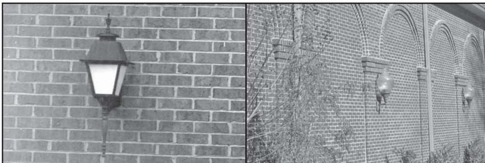
Lighting for nonresidential buildings shall not be residential in scale or design (left example). Such lighting shall be appropriately scaled to not overpower, or be diminished by the building. The right example is of appropriate lighting for a nonresidential building.
