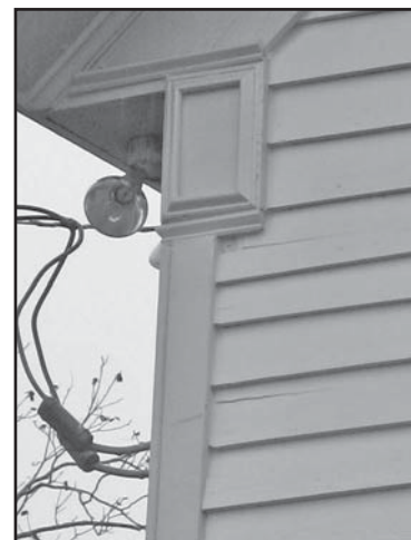
This chamfered corner board with elaborate cap is character-defining of this rehabilitated residence and was appropriately retained during the rehabilitation project.
