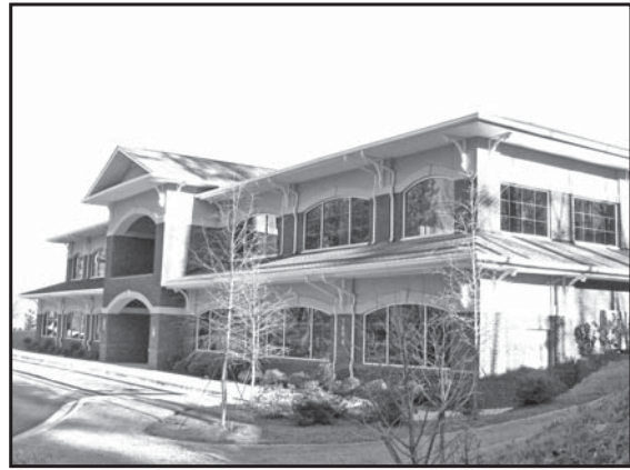
This commercial building features a uniformity of materials because the brick and stucco treatment on the front facade is continued on all primary facades.
