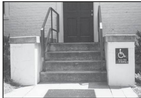
Signage that directs disabled persons to a less visible, yet accessible entrance, is a suitable design solution.
