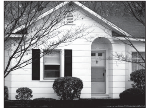
This recessed entry is a character-defining detail of this simple post World War II home on Old Highway US 41. The infill of this entry would be in appropriate.
