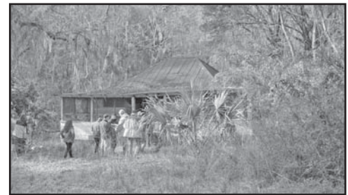
This cottage in south Georgia is an example of demolition-by-neglect.
