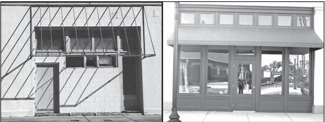
The Phoenix Hotel in Waycross, Georgia, was rehabilitated for reuse using the Secretary of the Interior's Standards for Rehabilitation . This project was part of both the Georgia and Federal Tax Incentives programs for rehabilitation. As part of this rehabilitation the storefronts which had been improperly infilled in the late twentieth century (see example above left) were remodeled to a more appropriate, traditional storefront design compatible with the rest of the building (see example above right).
