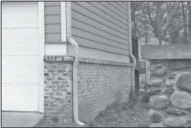
The use of a brick base with clapboard siding above on these exterior walls in Norcross, Georgia is an appropriate use of building materials to create architectural interest and would be appropriate in Kennesaw.
