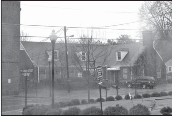
This commercial building is another example of a project adjacent to the historic commercial core of Kennesaw as well as the historic residential neighborhoods. This transition building utilizes the masonry construction of its nearby historic commercial buildings, while maintaining the residential scale (window size, shape and rhythm; dormers; and a chimney) of the adjacent neighborhood.
