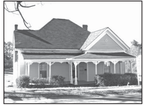
Traditionally gabled and hipped roofs were used within the district for residential construction.
