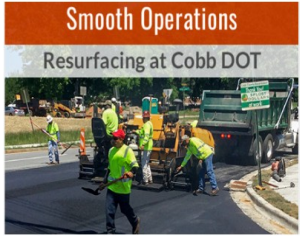
Smooth Operations: Resurfacing at CCDOT
